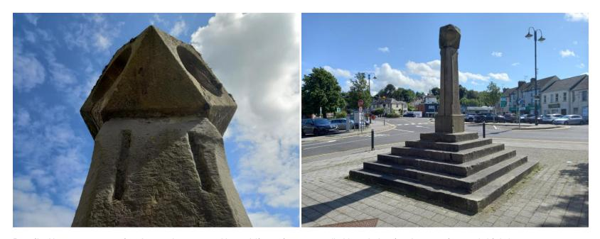
Detail of later augmentation for gas lantern and/or public notice mount (left) and chasing for gas pipework (right)
